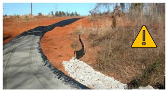
Geotextile keeps gravel from sinking into soft soil. Curving the road reduces the grade and gives room to install water diversions. Groundcover is needed on bare soil.
