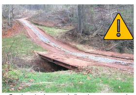
Good road using gravel, diversions, grass and bridgemats. Work is needed to level off the ruts and prevent sedimentation runoff into the stream.
