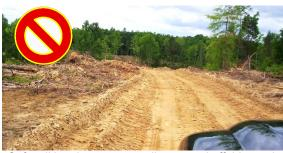
Soft soil has been repeatedly scraped off this road, creating side berms of soil that trap rainfall runoff. Significant regrading is needed to reshape this road.
