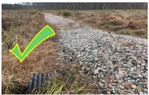
This wetland road is low profile, has gravel and uses a cross-drain pipe to allow water to equalize on both sides.
