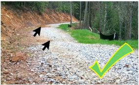
Broad-based dips are built in the road (arrows). There is ample gravel and the road edge is stabilized with grass.
