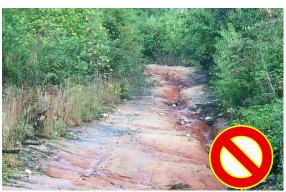
An erosion gully is carving away the road because it lacks water diversions and surface stabilization.
