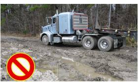
This road is sloppy and has lost its structural integrity. Sedimentation into streams is very likely and extra wear and tear on equipment is possible.
