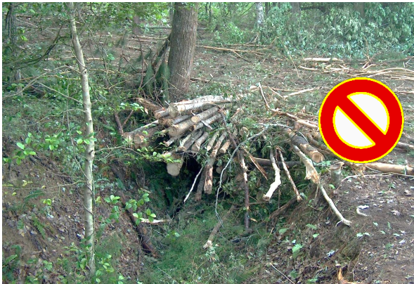
Pole crossing in a dry ditch for haul road access.
