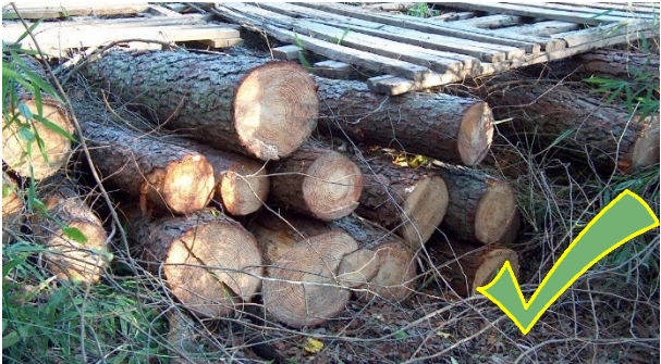
Pole crossing in a dry ditch for haul road access.
