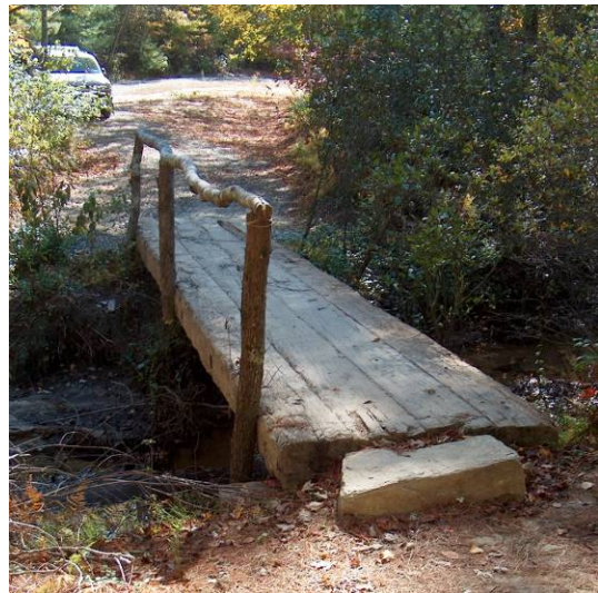
Figure 7: Retired bridgemat used on a hiking trail.
