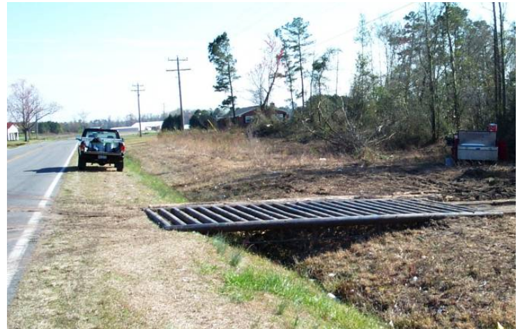
Figure 12: Duplin County, 2001. This open-grid bridgemat panel allows log trucks to cross a DOT roadside ditch. Not only does this bridgemat avoid the need of filling in the road ditch with a culvert or with logs, but the open-faced configuration helps to 'shake off' any caked-on mud from the truck's tires prior to entering the public roadway.
