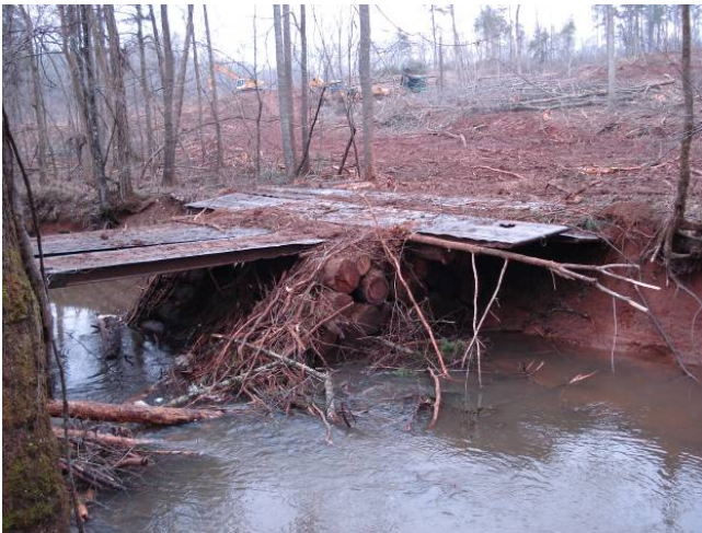
Figure 3: The logger used NCDFR bridgemats for the center span on this crossing and used his own bridgemats on the approachway.
