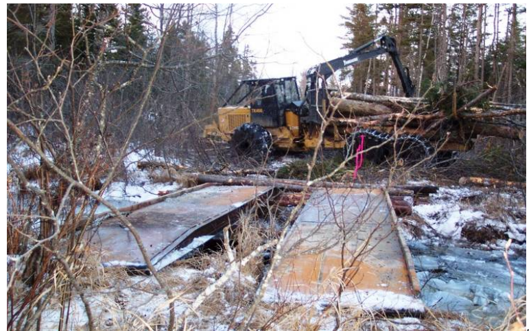
Figure 10: Maine 2007, photo provided by Maine Forest Service. Note that their bridgemat design also includes side-rail guards, but of a different configuration than those seen in the photo at left.
