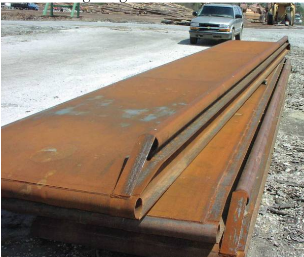
Figure 9: Wayne County, 2003. Note the side-rail incorporated into the bridgemat. Installing a side-rail guard will limit where or how each panel can be positioned over the crossing, since there is now a definite “inside” and “outside” of each bridgemat.
