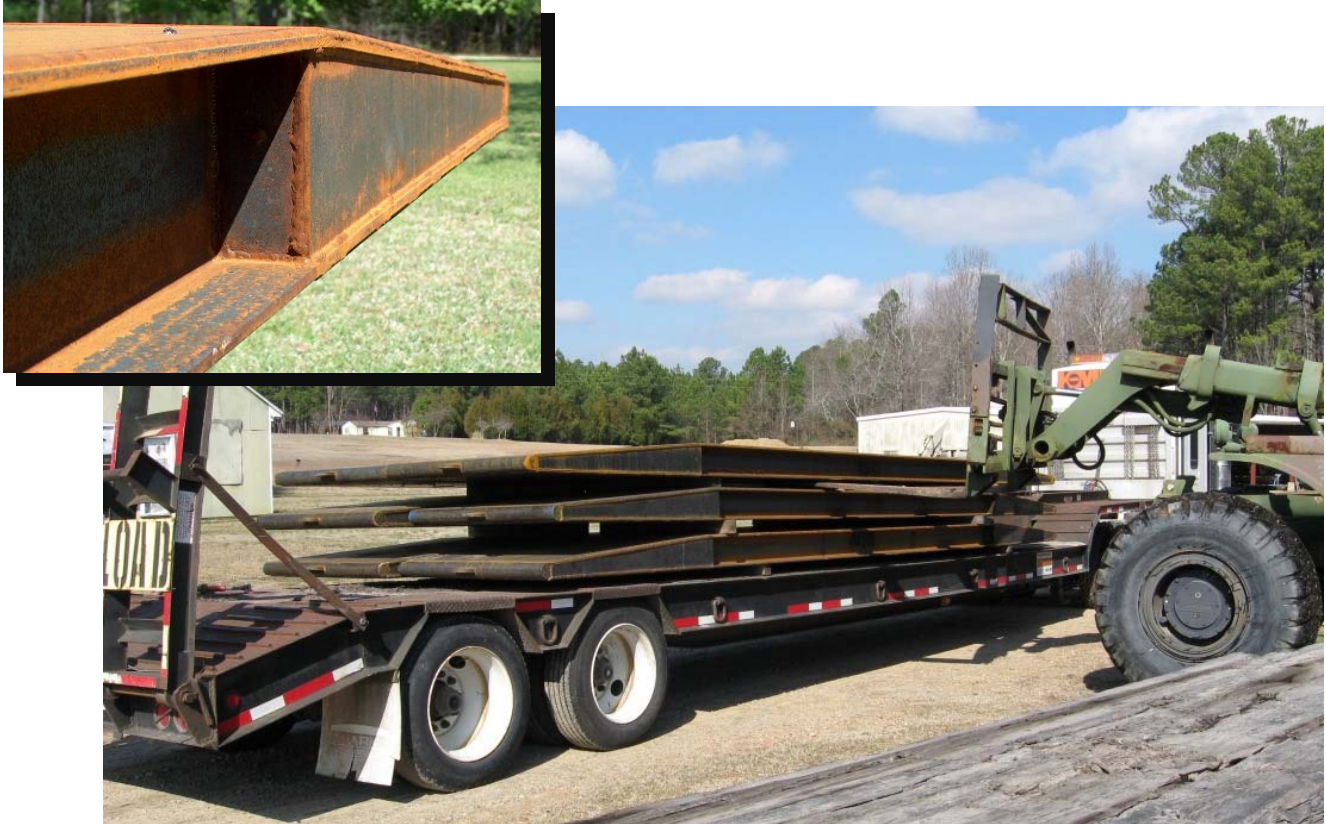
Figures 15 and 16: Johnston County, 2008. A shipment of new, 25-foot long steel bridgemats is received by the NCDFR and being unloaded for staging. On this bridgemat order, the addition of a steel plate along the sides of each end-ramp of the bridgemat was specified, effectively boxing-in this area within the I-beam flanges (see inset photo, above left). This is an attempt to strengthen the end-ramps and reduce the crimping damage we have observed when a grapple-skidder grabs the end for handling or moving the bridgemat. The addition of a boxed-in end-ramp may also increase the rigidity of the bridgemat.
