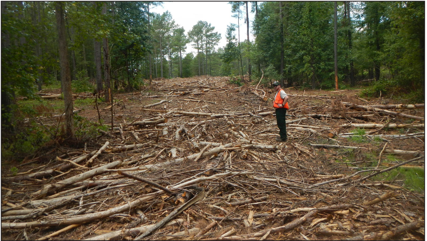
Photo 11. This main skid trail has ample logging slash (laps) applied atop of the ground surface. When applied at the onset of the harvest, and frequently added to, this material provides instant groundcover protection of exposed soil and reduces impacts to the soil.
