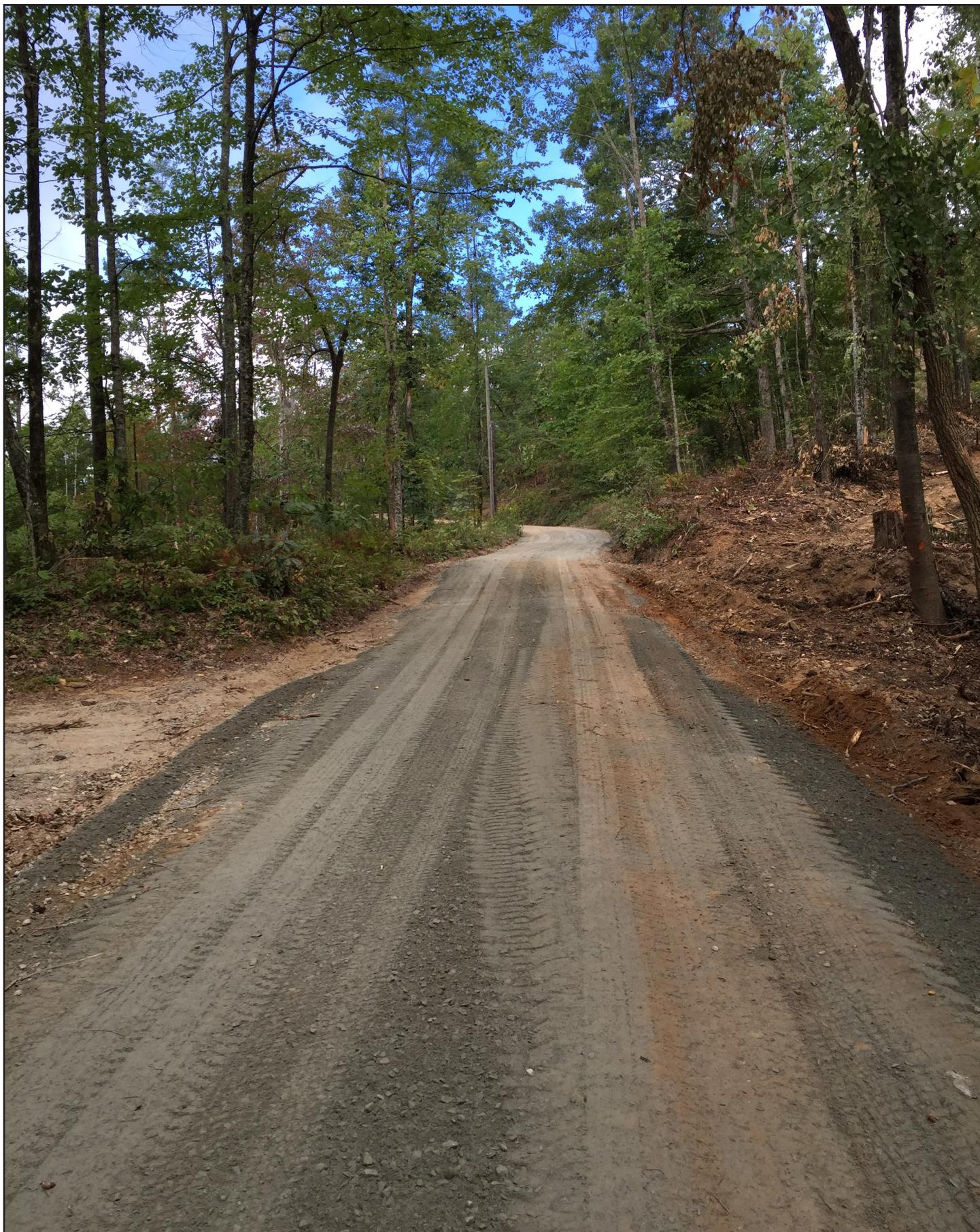
Photo 15. A well-maintained forest road. A shallow broad-based dip or similar water diversion is visible near the top of road. On sloping sections of road, it is important to frequently install diversions to control runoff and capture sediment before it can reach a waterway.
