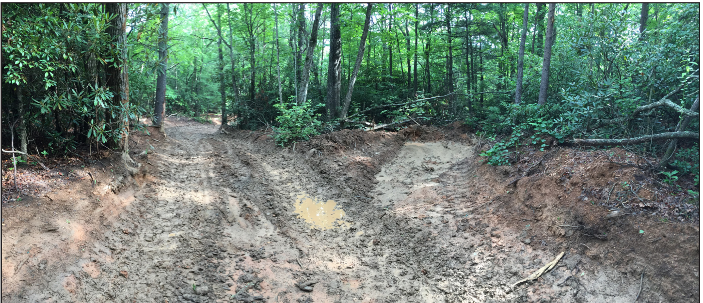
Photo 1. Though equipment traffic over this wet soil has the potential to cause rutting, the operator installed periodic turnouts on this skid trail to capture runoff, as seen on the right side of the skid trail.
