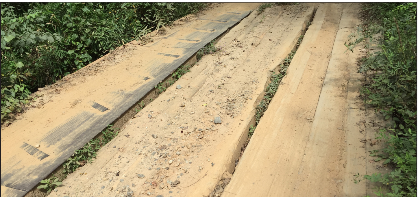
Photo 17. Though the use of bridgemats is recommended, they must be used correctly. Bridgemats must be tightly bunched together to limit gaps between them as much as possible. In the current arrangement, sediment can wash through the gaps between the mats, and enter the stream.
