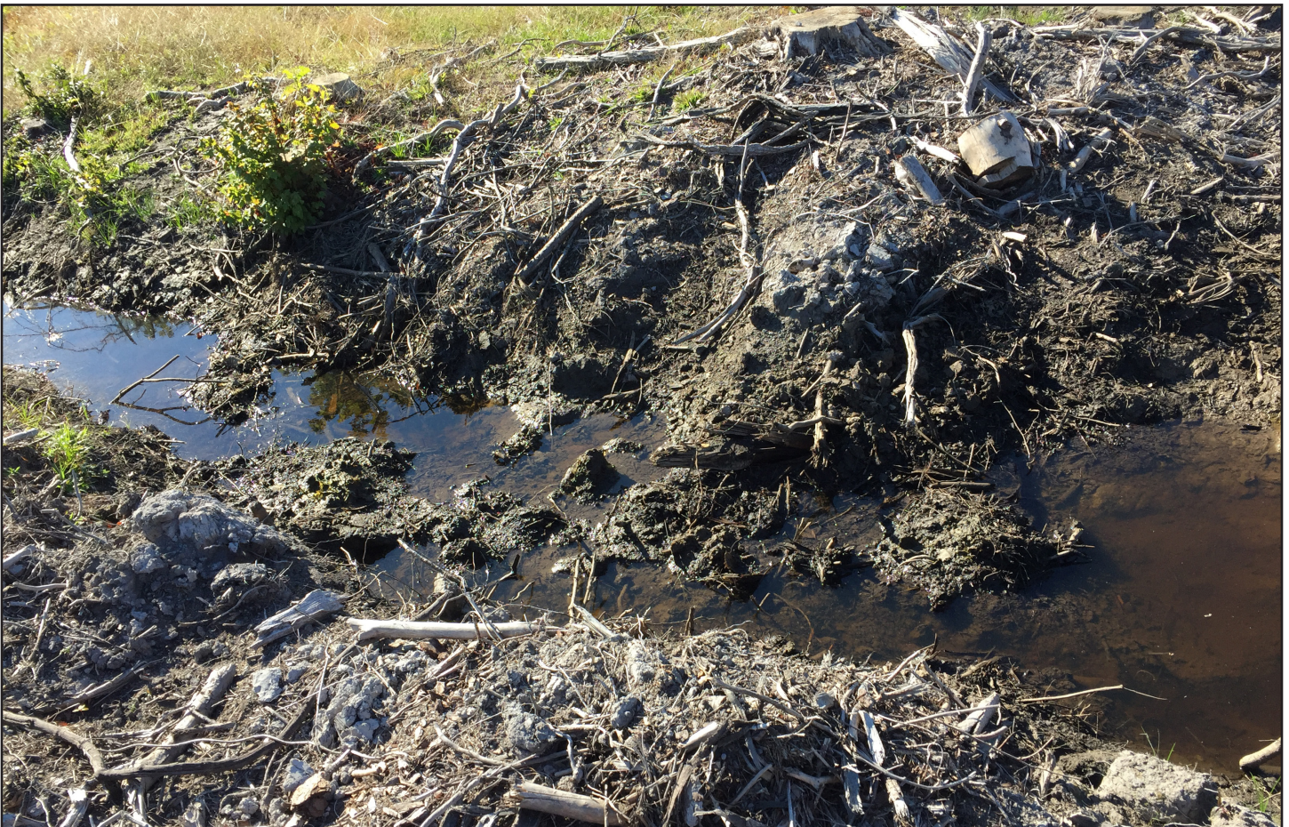
Photo 19. On this crossing in the Coastal Plain, it appears that skidders traveled directly through the waterway, disturbing the banks, and dragging sediment and debris into the waterway. This was characterized as a ford crossing by our evaluators. Fords should not be used on skid trails. A bridgemat would have likely been the best option in this example, or perhaps a temporary culvert crossing.
