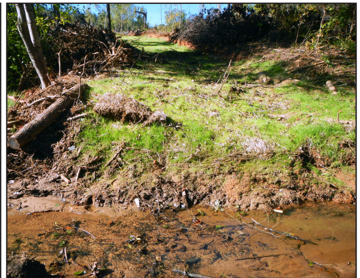
Photo 10. A properly stabilized stream crossing with ground vegetation established and water diversions installed.
