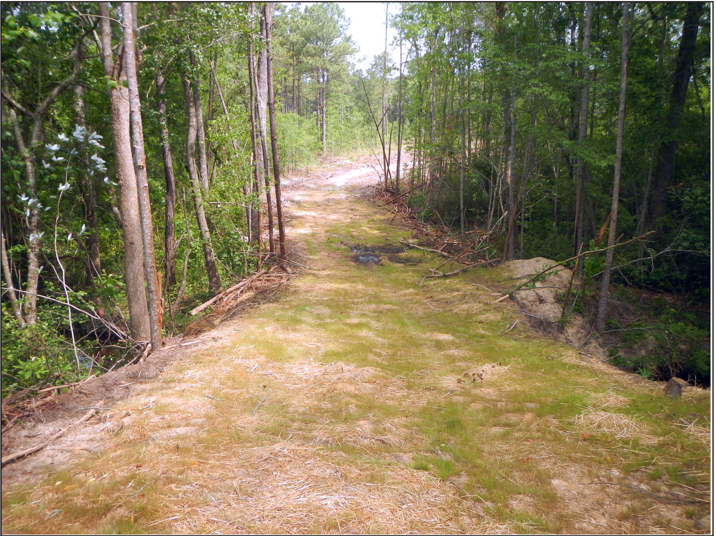
Photo 8. This roadway through a SMZ has new vegetation emerging that will stabilize the soil.
