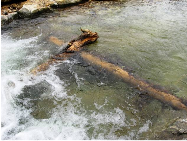
Photos above show close-up of woody material that was incorporated into the design. Top-Left: A log X-vane was installed within one of the pools, below a rock/boulder vane structure. Top-Right: Bundles of small woody material were partially buried in sections of the new streambank.
