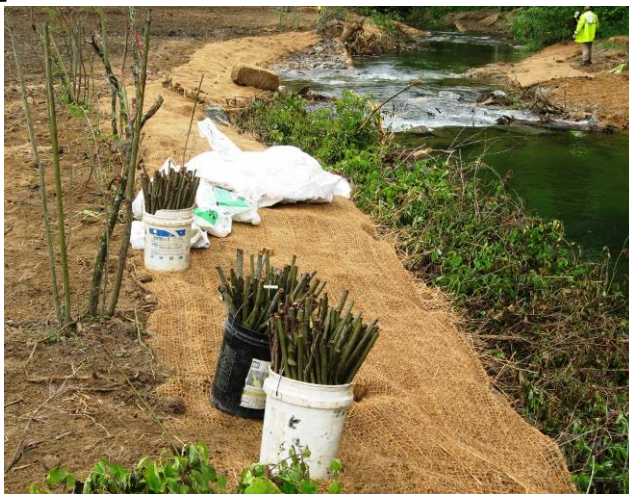
Photos above show steps taken for streambank and groundcover stabilization. Top-Left: Live stakes to be installed, and coir matting already installed. Top-Right: Straw is blown across the area after grass seed has been applied.
