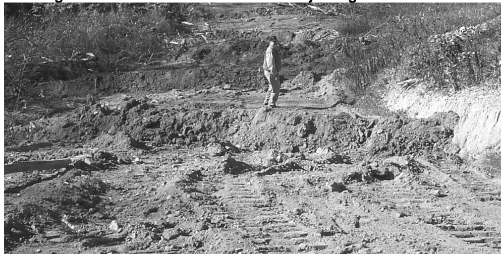
Figure 5D: A waterbar tied in to the adjoining side / cut bank
