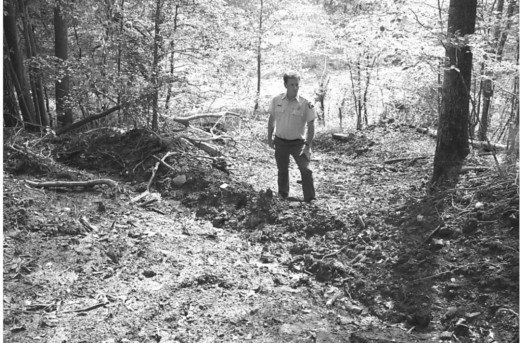
Figure 5B: Waterbar constructed across a skid trail in Wilkes Co., N.C.
