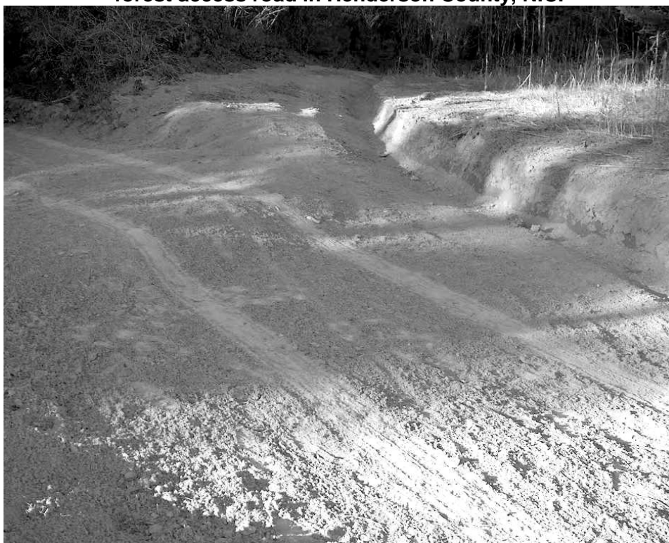
Figure 5F: A turnout, used as a wing ditch alongside a forest access road in Henderson County, N.C.
