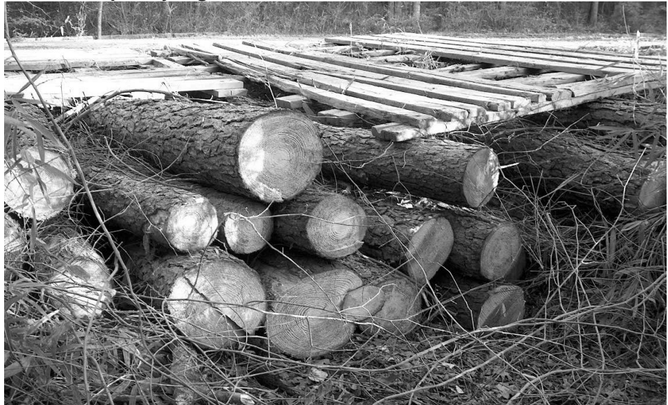
Figure 5Z: A pole crossing installed within a dry ditch for temporary log road access in northeastern North Carolina
