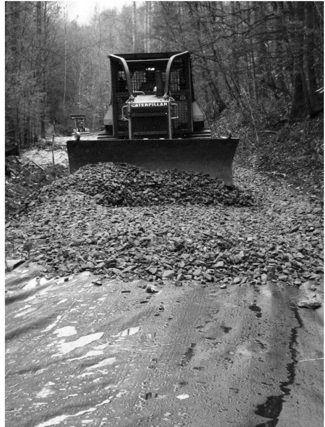
*Photos of geotextile underlayment and stone aggregate applied atop a freshly-graded forest road on
