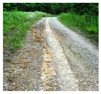
This road needs re-grading, installation of water control diversions, and significant groundcover establishment work.
