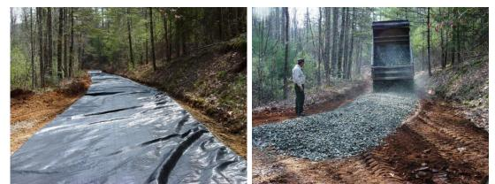
Geotextile filter fabric installed on the left, and gravel being applied atop of the geotextile on the right.
