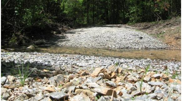
This ford crossing was installed to replace an improper crossing of logs, boulders, and soil. The stream is now open and free to flow, without excessive fill material blocking the channel.
