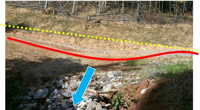
This is a side view of a broad-based dip. The dotted line shows the original road grade. The curved solid line shows the new, gently rolling grade of the roadbed. Runoff that flows off of the road surface will exit the broad-based dip atop of the large stone.
