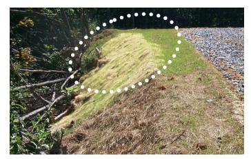
This matting is made from small fibers of wood, straw or coconut husks. It works well to stabilize and create a seeding foundation upon slopes, within roadside ditches, and along stream banks. Erosion control matting should not be used in a location where vehicle traffic is expected. Do not drive over the matting. Apply lime, fertilizer, and grass seed prior to laying down the erosion matting. Firmly anchor the matting
