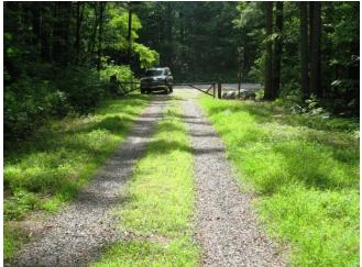
The minimum width of the roadbed should be 14 feet wide for one-way traffic and 20 feet wide for two-way traffic. The minimum tread width is 10 feet for one-way traffic and 15 feet for two-way traffic.
