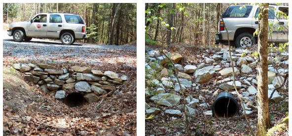
These two photos show the same cross drain culvert through a curve in a road. The culvert is placed within a dry gully that only carries water after rainfall. The photo at left is the uphill inlet end. The right photo is the downhill outlet end. Each headwall is armored with native stone obtained on the property -- a good way to save money!
