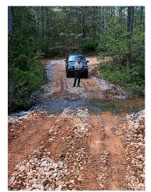
This ford crossing needs work. Gravel is getting pushed into the soft ground. Mud is being pulled into the creek.
