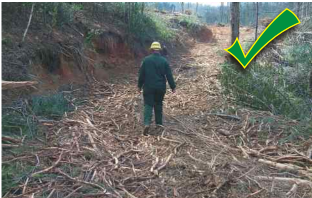
Brush is packed down on this skid trail to control runoff.
