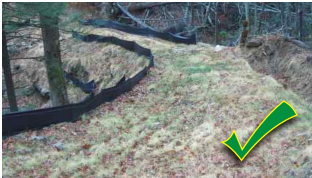
Skid trail is closed-out and stabilized
