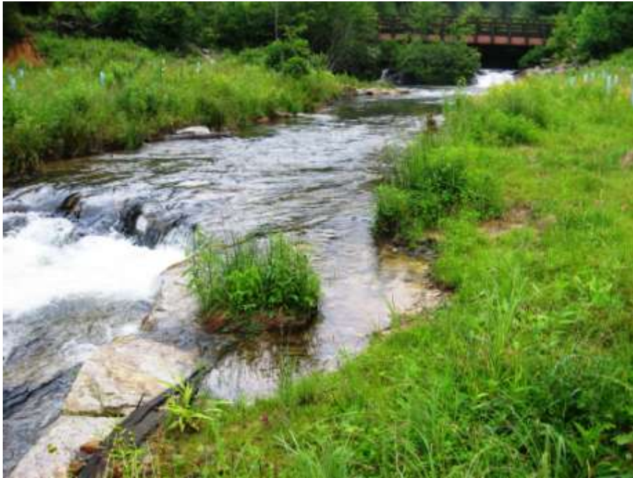
Photo above in July 2013: The stream repair has stabilized and vegetation is re-colonizing the area. The stream flow seen here is near bankfull after steady, heavy rains in the region over a period of days in late June and early July.
