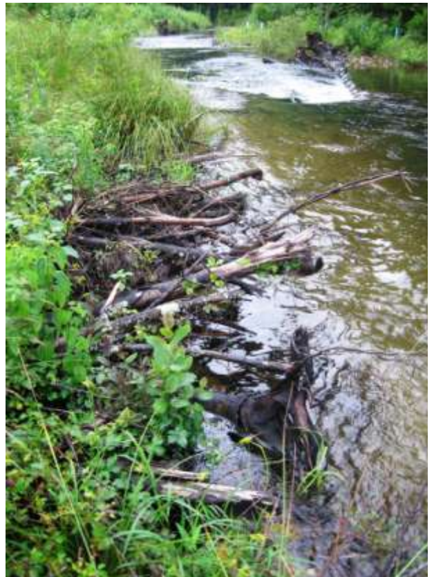
Photo Right, July 2013: Brush toe material on left bank remains intact and functioning, seen here at bankfull, or near bankfull.
