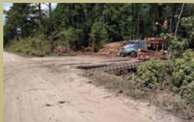
**Above:** Bridgemats and logging mats installed over a roadside ditch.
