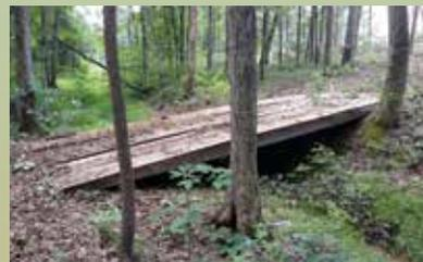
**Left:** A set of properly installed bridgemats protecting the stream channel;
