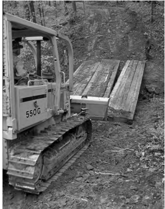
Dozer aligning bridge panels across an intermittent stream in Eastern Kentucky
