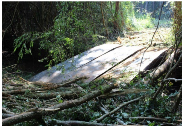
Figure 1 Temporary bridge in use on an active forest operation.
