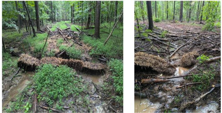
A closed skid trail shortly after a rain event where straw bales were used to help reduce sedimentation at two different stream crossings.
